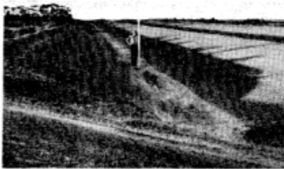
A road grader can leave a catchment surface smooth and with uniform road side—slopes, but final catchment surface preparation should be done with a heavy roller with the soil at or near optimum moisture content for compaction. The best surface for promoting runoff results from compaction with a 6 tonne multi—tyred road roller. Six passes of a roller with the soil at optimum moisture content will give a good surface, and this will usually amount to 4 hours of rolling per hectare.
