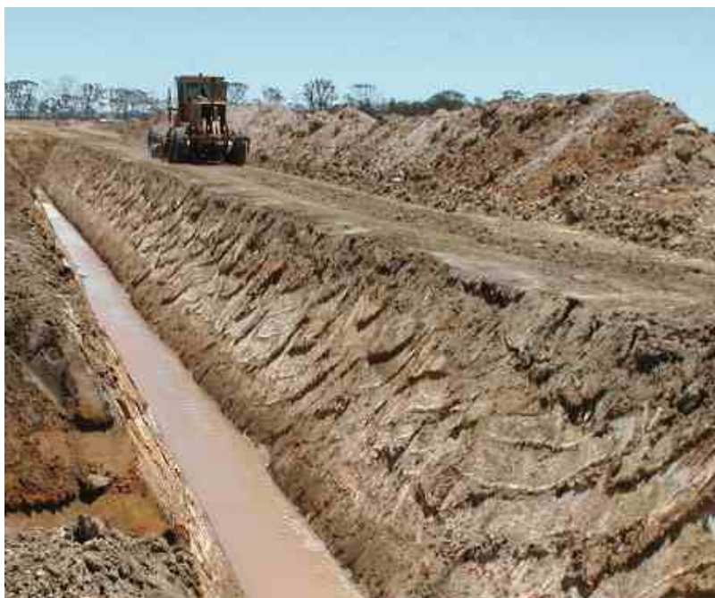
A wide berm between the drain and spoil bank allows machinery access for maintenance.
