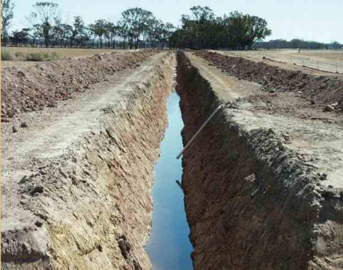
*A double leaved deep drain with surface water inlet pipe. Surface water can be drained from outside the spoil bank by piped inlets that extend through the bank at ground level and discharge into the drain.*
