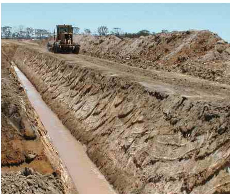
*A wide berm between the drain and spoil bank allows machinery access for maintenance.*
