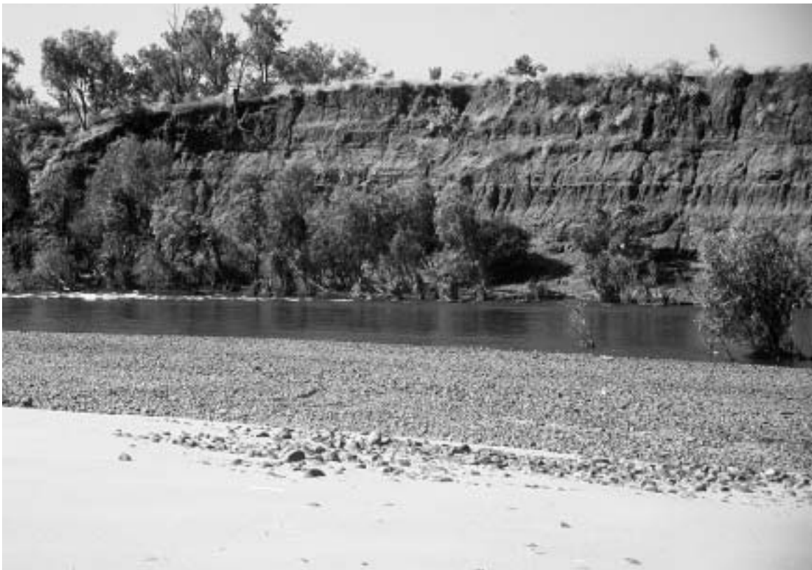
The Ord River cutting into levee soils adjacent to the survey area near Button's Crossing.
